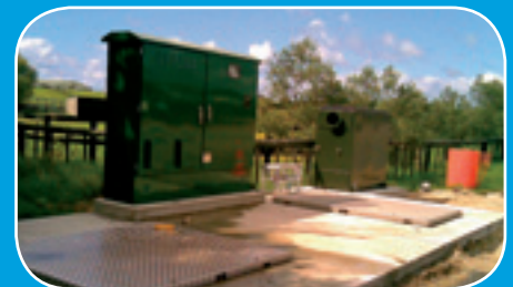
Ruakaka Wastewater Upgrade
